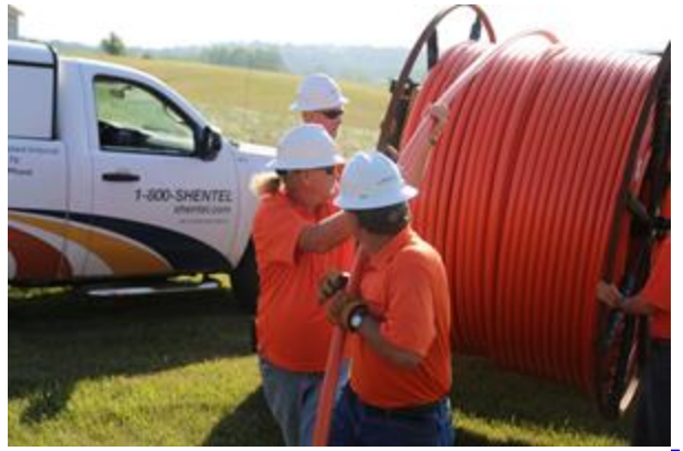
Shentel construction team running reels of new fiber line.
